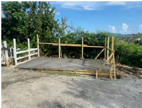
Concrete pad for garbage bin enclosure
